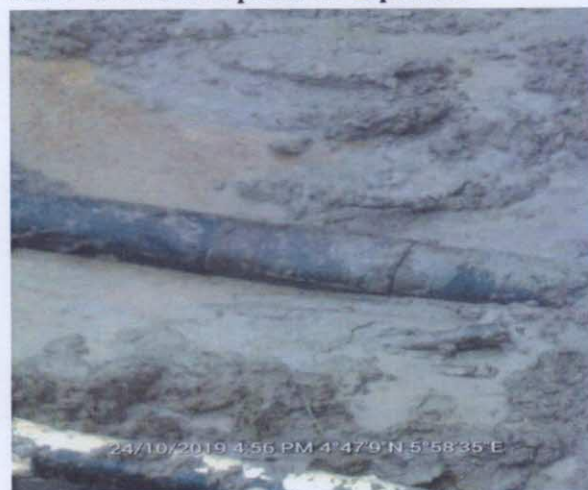
FIG E-F: Incident point after repairs
